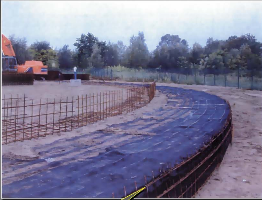
Reinforced earth wall
